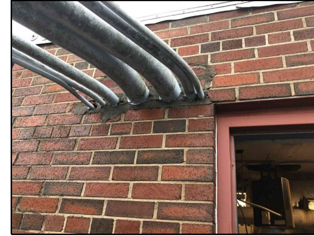
5 CONDUIT PENETRATION AT EAST GYMNASIUM PARTITION
