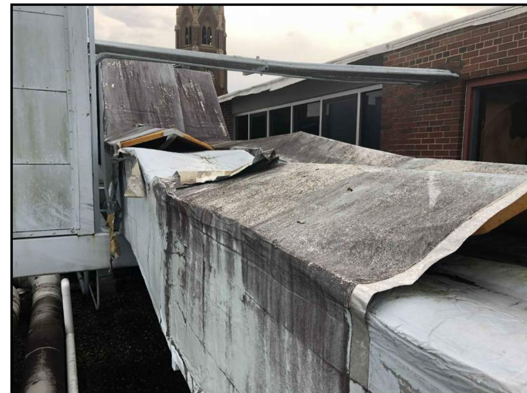
13 DAMAGED DUCTWORK AT GYMNASIUM
