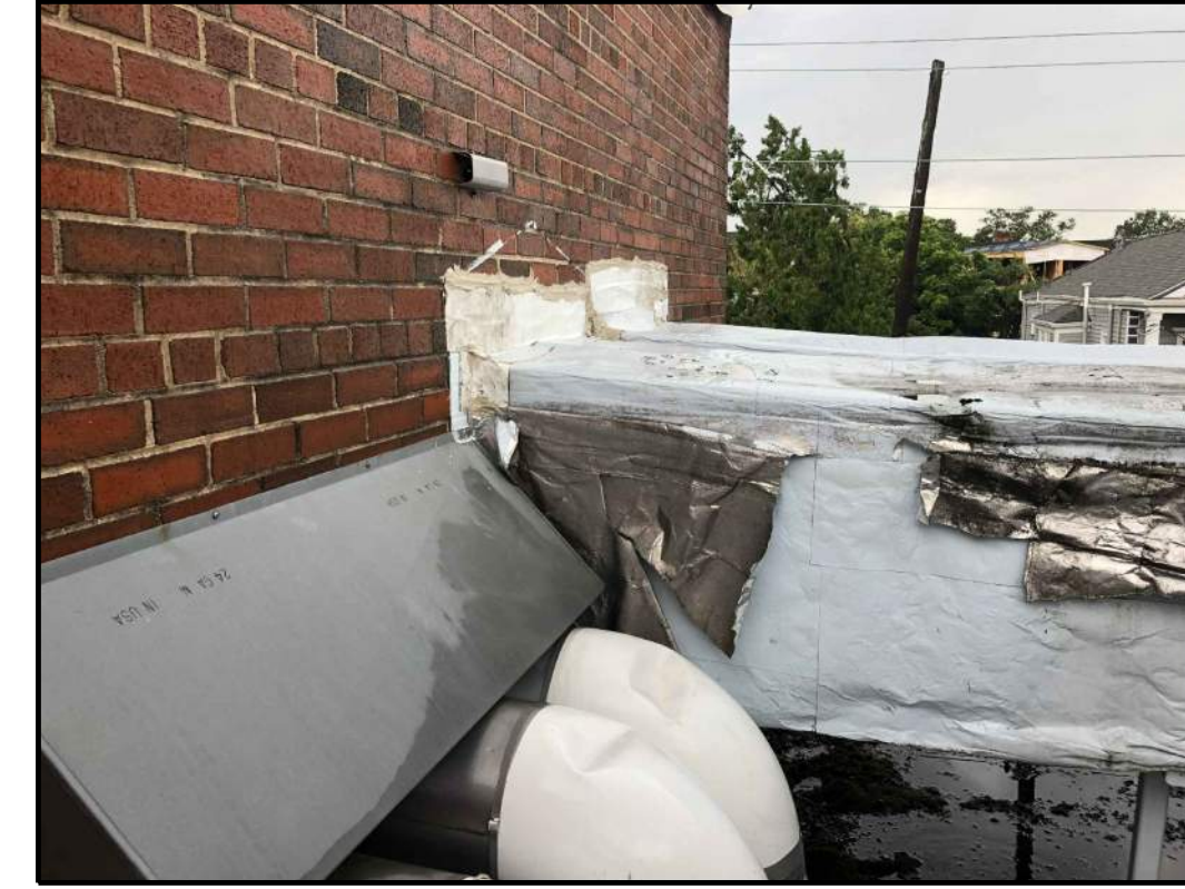
4 DUCTWORK AND CHILLED WATER PIPE PENETRATION AT EAST GYMNASIUM PARTITION
