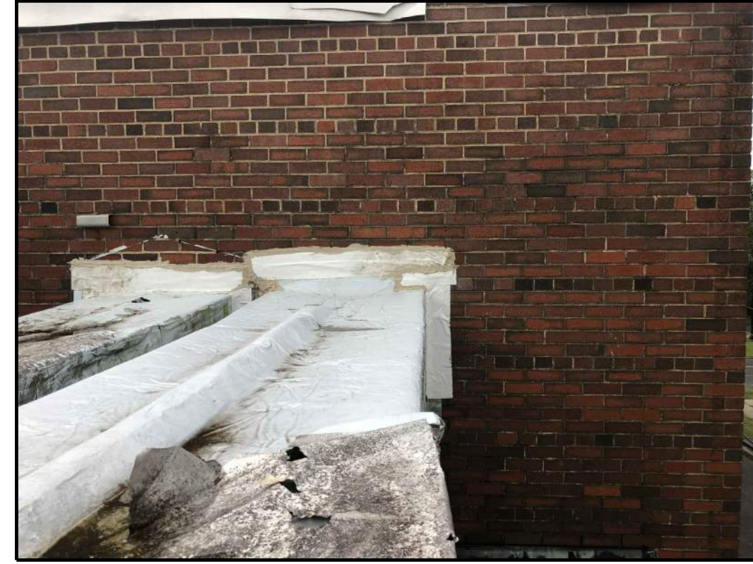
3 DUCTWORK PENETRATION AT EAST GYMNASIUM PARTITION
