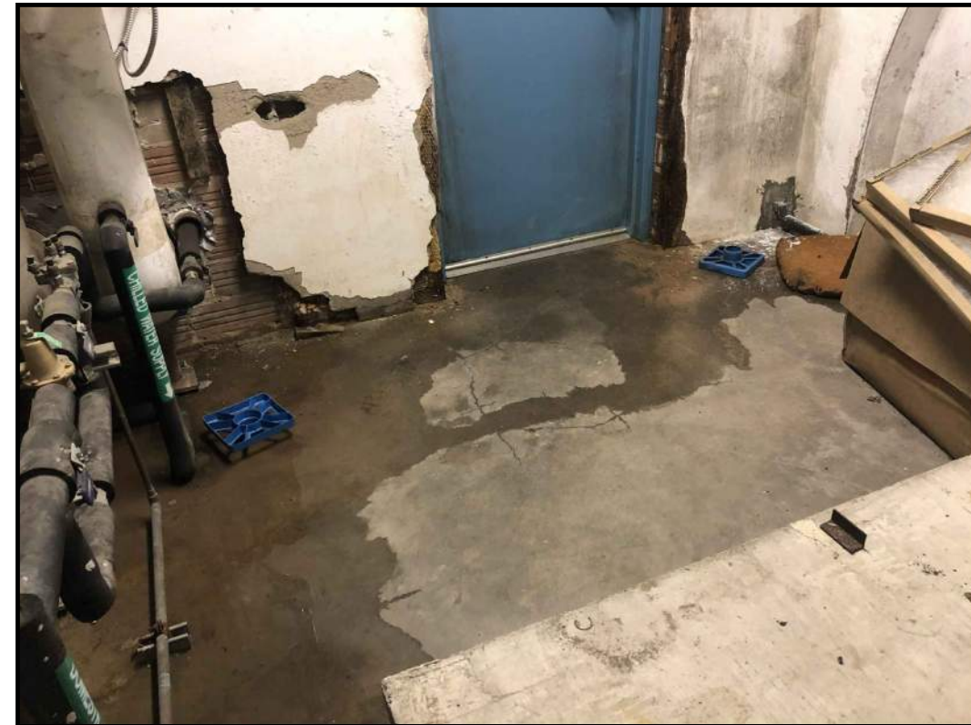
7 PLASTER SPALLING INSIDE MECH. EQMT. ROOM
