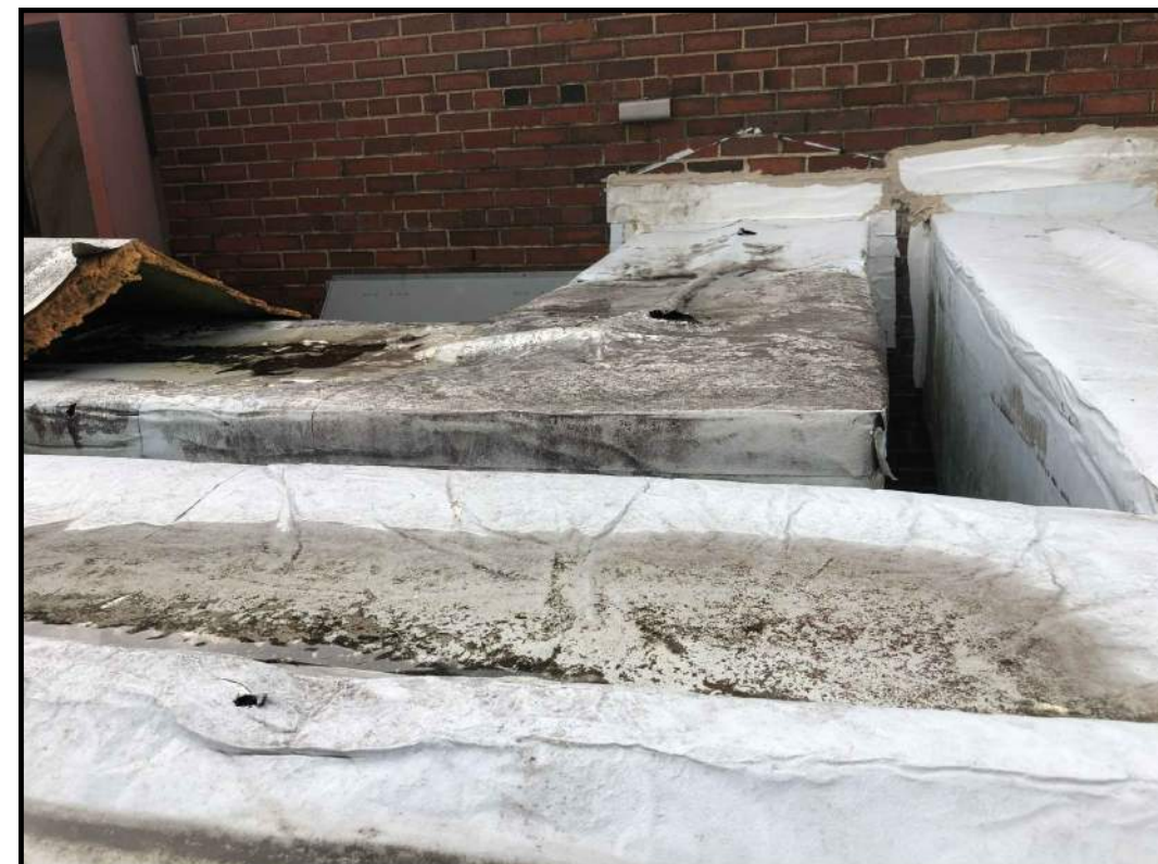
12 DAMAGED DUCTWORK AT GYMNASIUM
