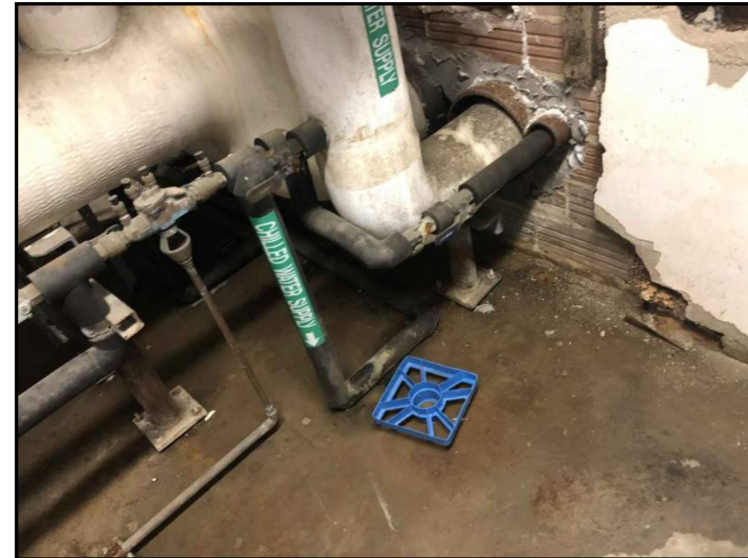
8 PLASTER SPALLING INSIDE MECH. EQMT. ROOM
