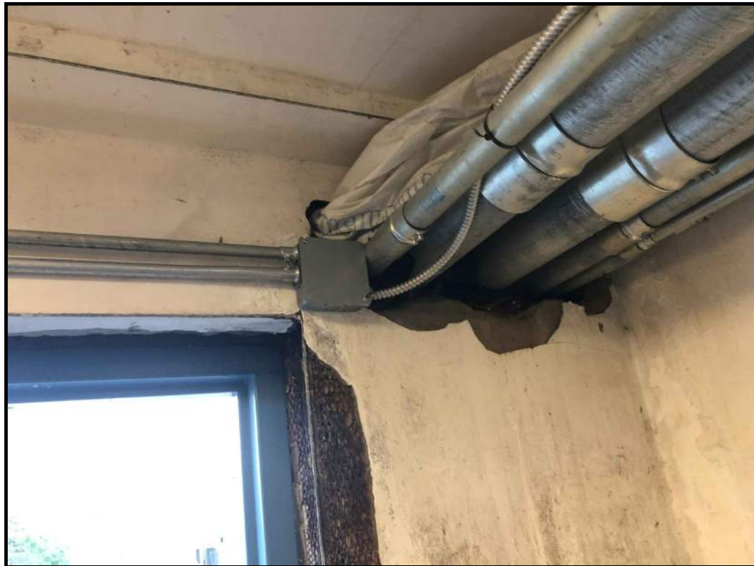
6 CONDUIT PENETRATION AT EAST GYMNASIUM PARTITION
