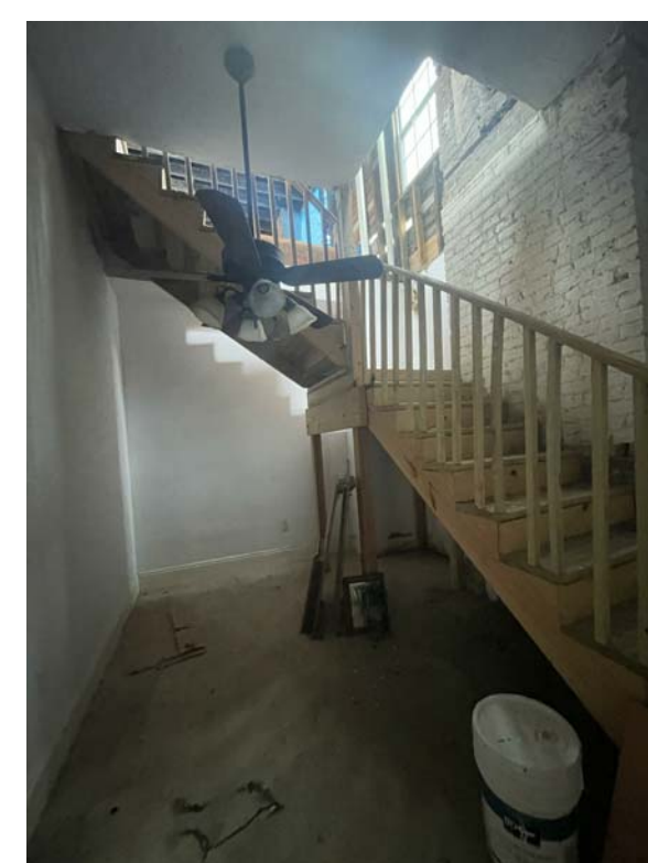
Existing stair to unit 2
