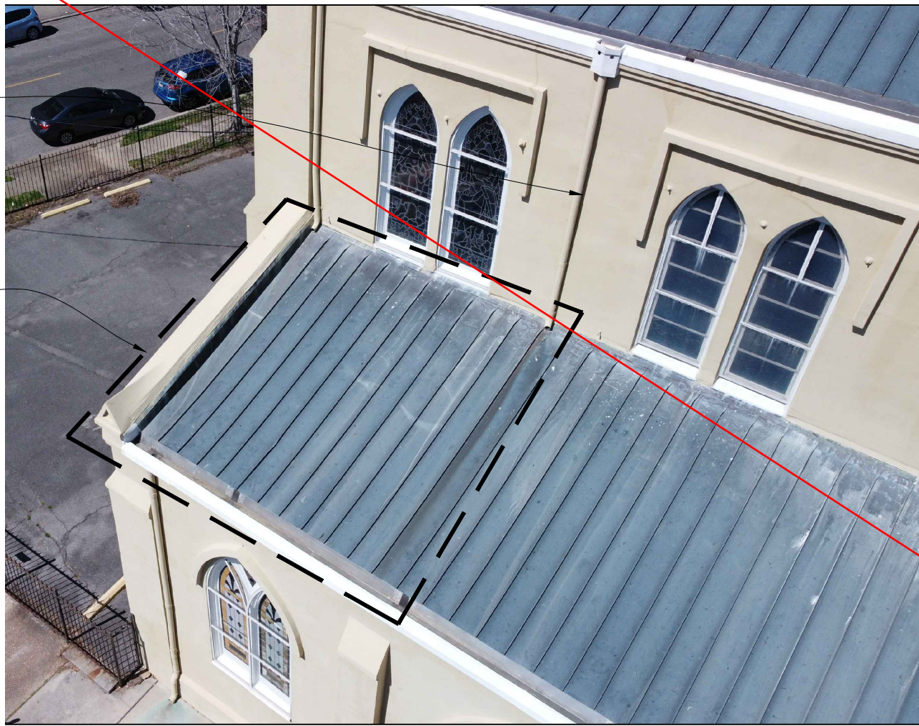
3 STANDING SEAM JOINTS AT REAR OF CHURCH A1.01 SCALE: N.T.S.
