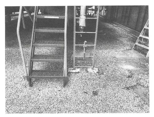
At the three ladder/stair locations on this roof area, none of these penetrate the existing roof system. Assuming space exists, we propose to install Siplast's Paratread walk pad beneath each footing. On top of the walk pads at each stair/ladder support, we will then install an aluminum plate in order to more evenly distribute the load if pressure is placed on the roof system while these items are in use or if they settle over time. The size and thickness of the plates are to be determined.
