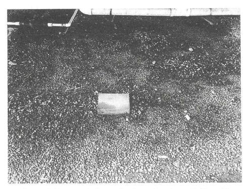
At least two flashing penetration boxes, such as the one shown above, exist. These will be replaced with new stainless-steel flashings with tops, or these can be eliminated. Electrical, mechanical, and related items are excluded from this Proposal.
