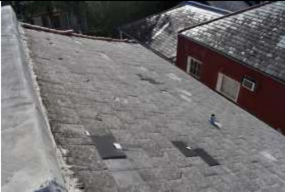
Main Roof - Left
