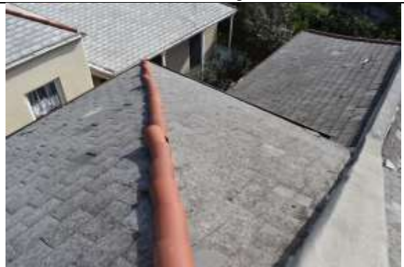
Main Roof - Hip Right Rear
