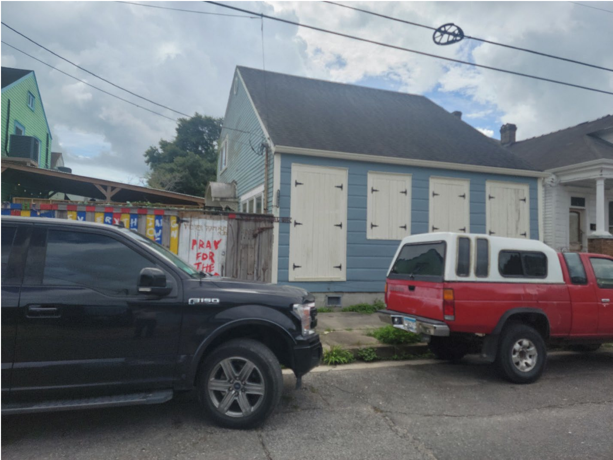
Photos from Piety Street. 2-story “salt box” structure obstructs much of the view of the proposed covering.
