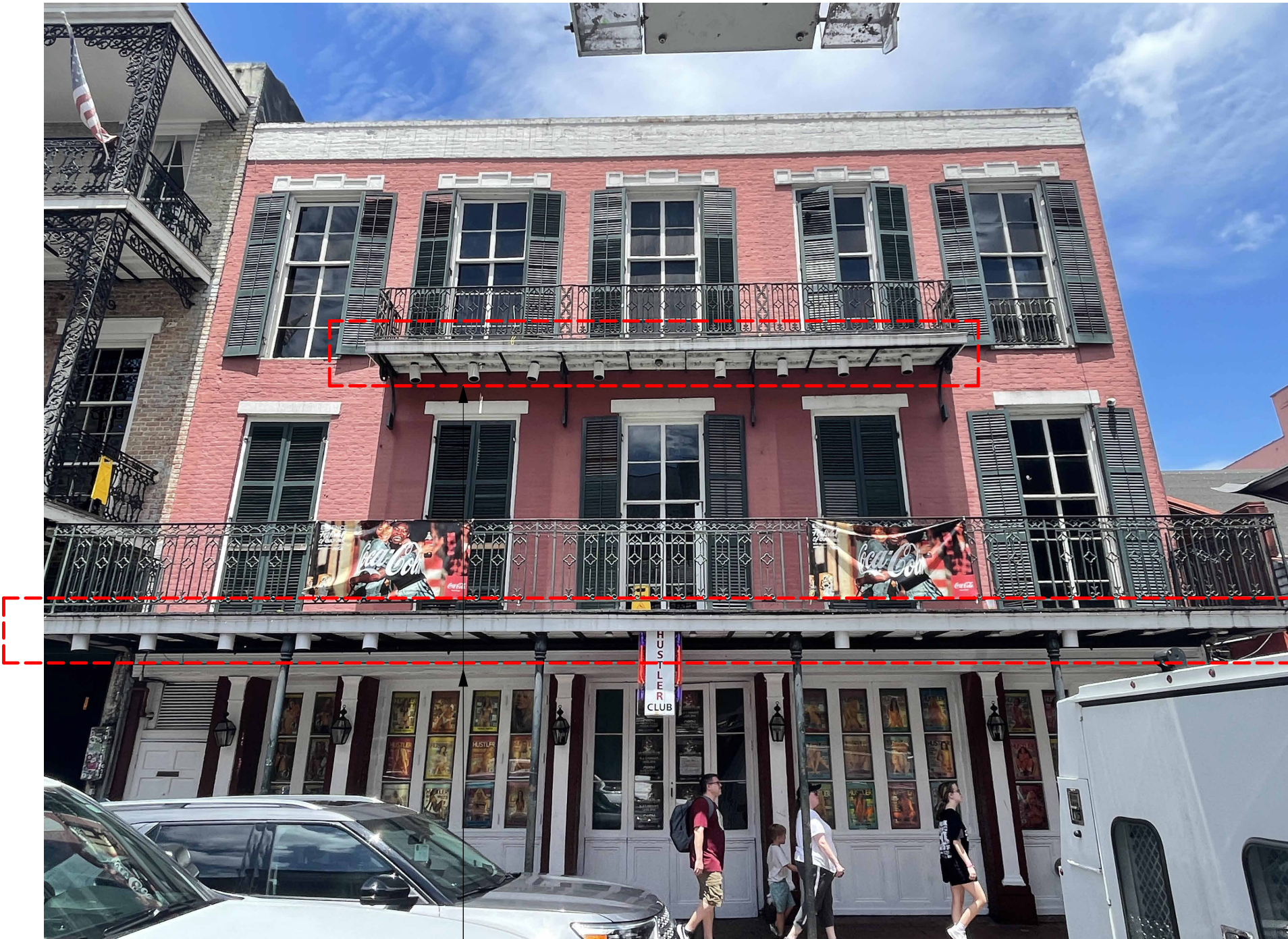
LIMITS FOR SCOPE OF WORK. REPLACEMENT OF DECKING ON 2ND FLOOR BALCONY AND 1ST FLOOR GALLERY
