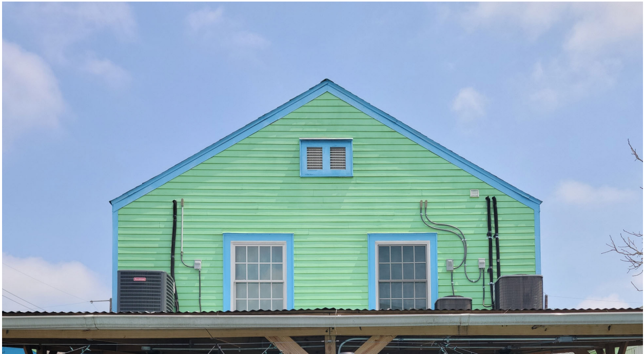
REAR GABLE AT EXISTING MAIN BUILDING ON SITE
