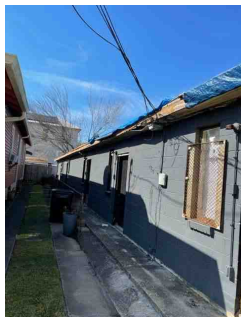
Rear Yard / Shed
