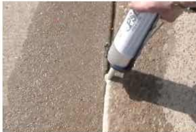
E-101 Applied To Wet Concrete
