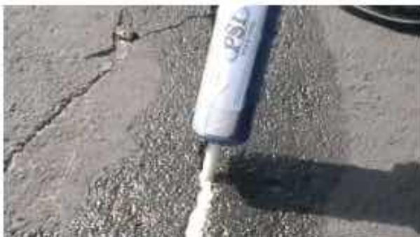
E-101 Applied to Wet Asphalt Cracks
