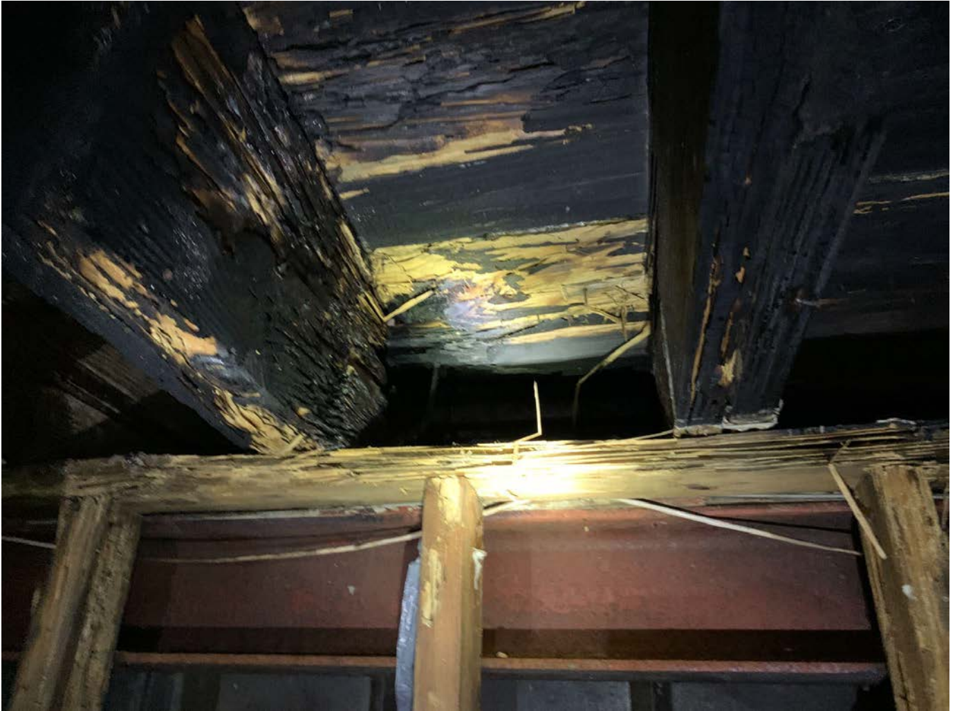
Charred ceiling joist with old termite damage
