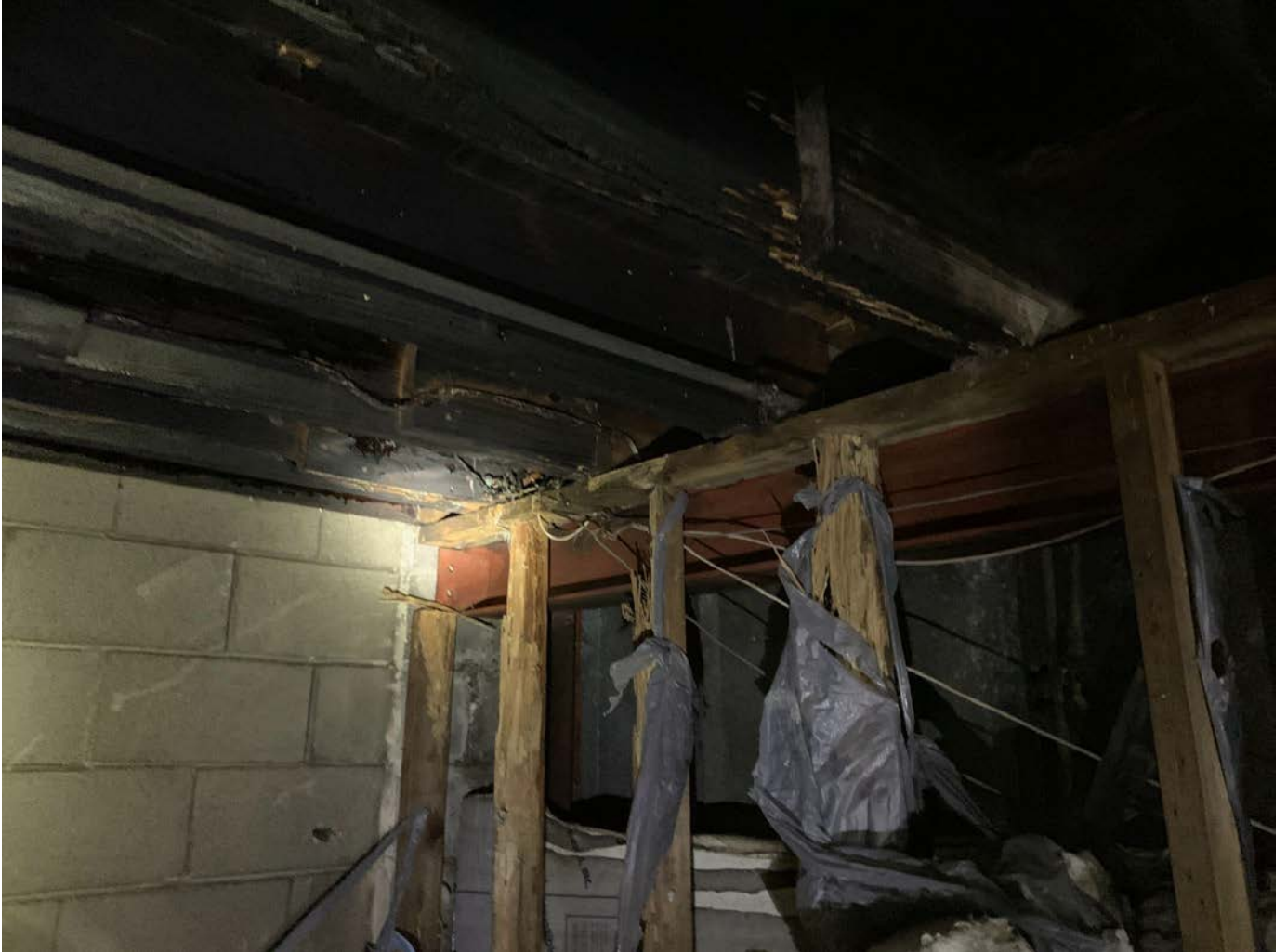
View of charred joist at front
