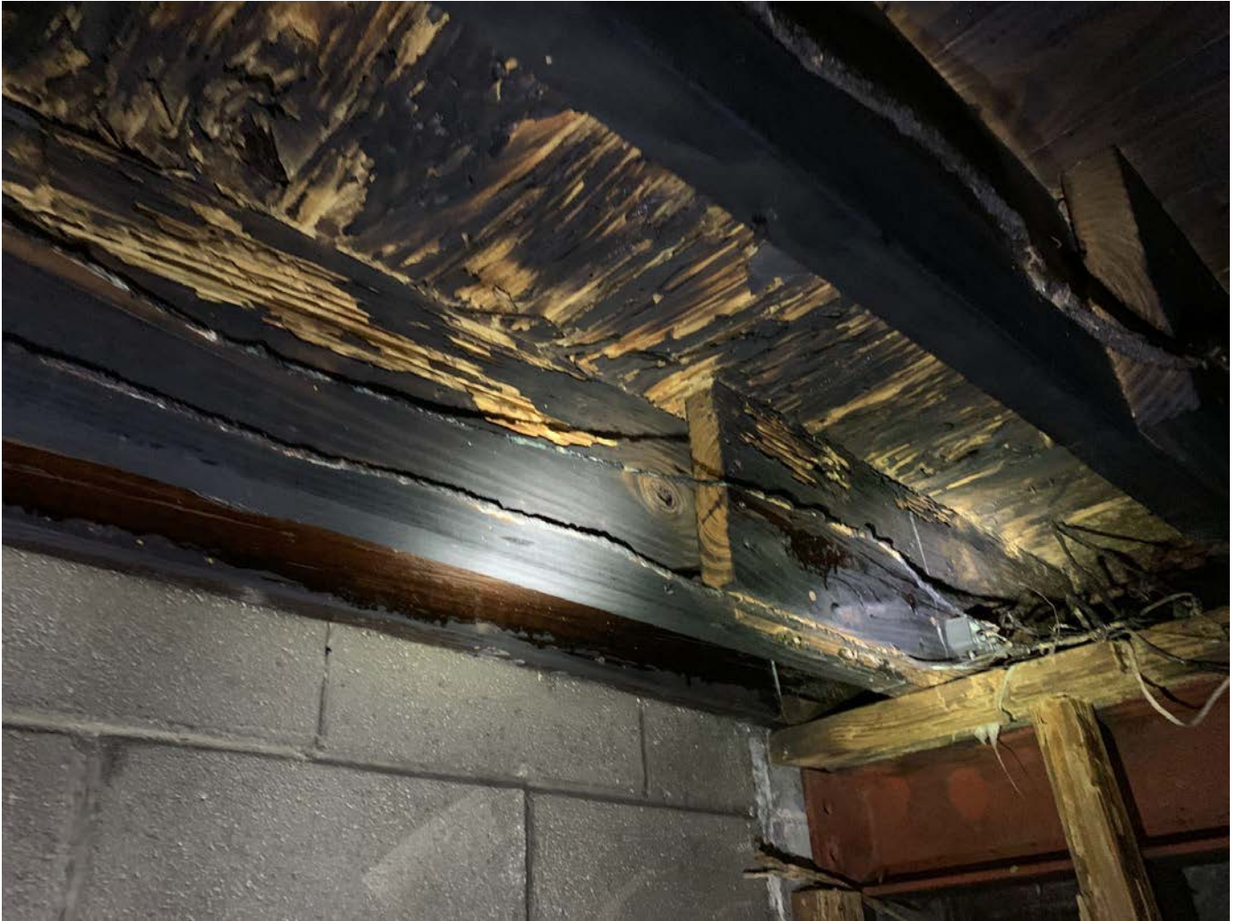
Charred subflooring, joists and termite damage
