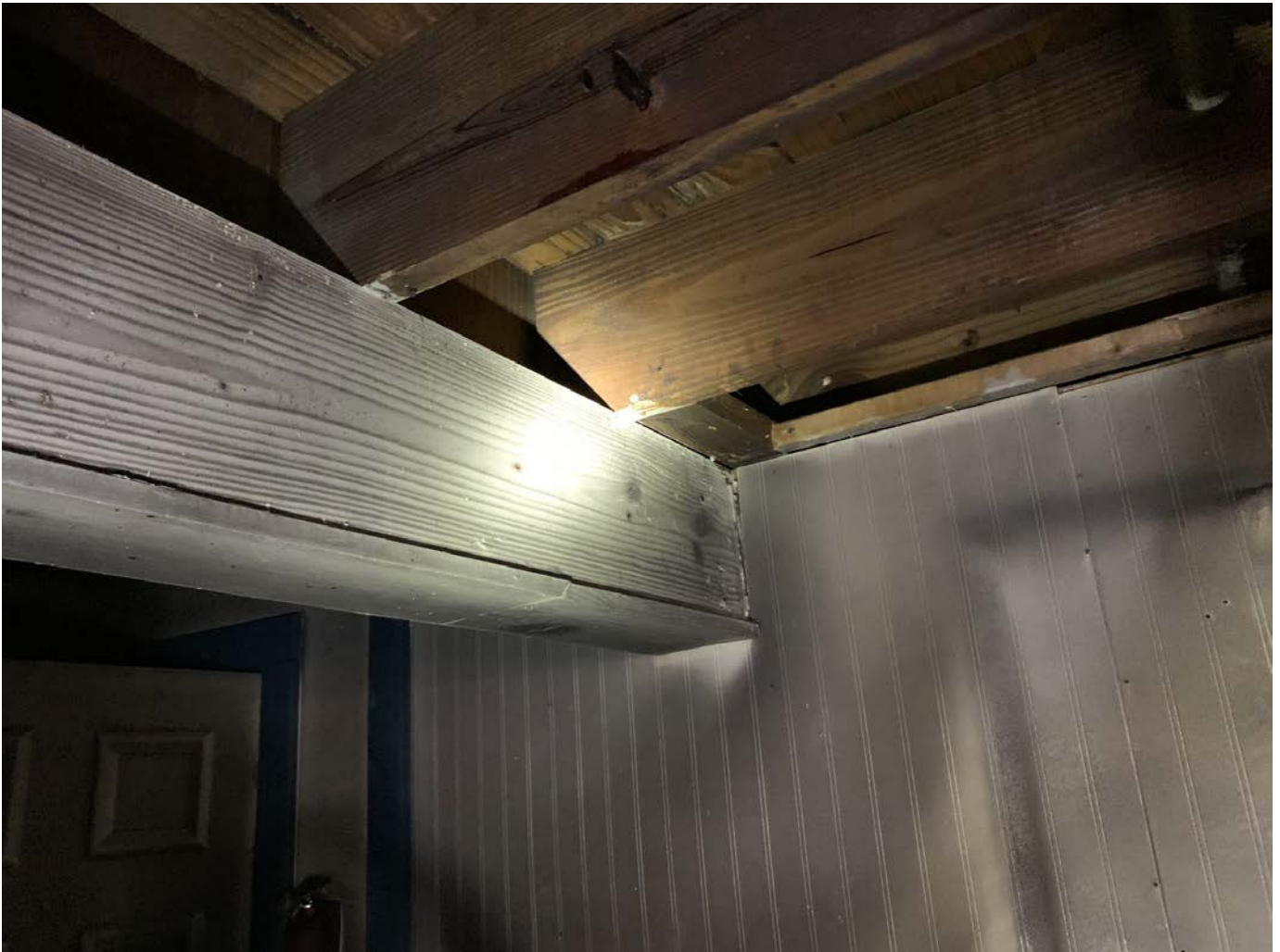
Beam supporting joists in rear of tasting room was undamaged
