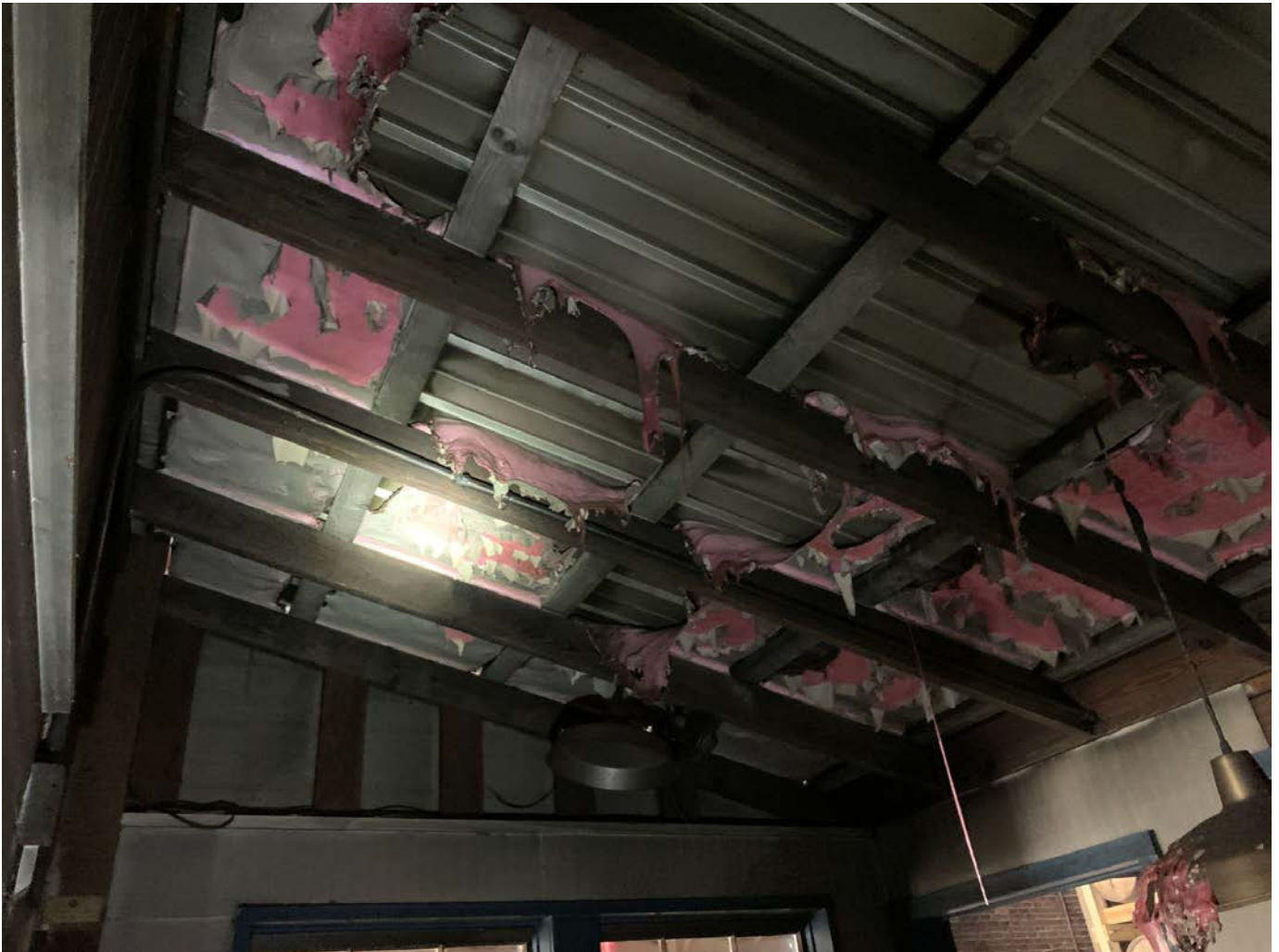
Smoke staining to rafters at rear of tasting room which were undamaged
