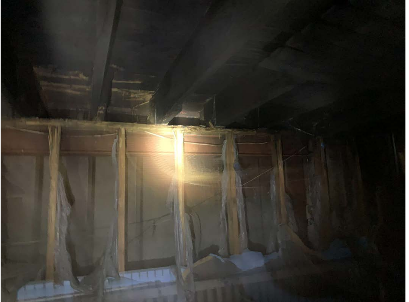
View of charred ceiling joists in tasting room
