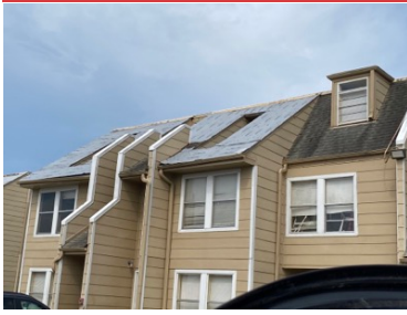
BUILD 15 2nd roof area
