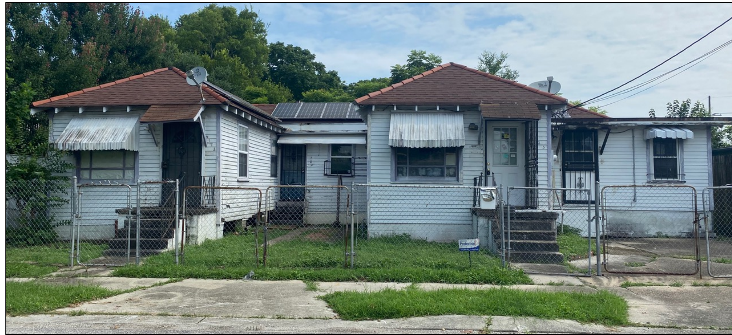
1 G-1 Photo of Existing House: View from Marais Street. Scale: 1/8" = 1'-0"
