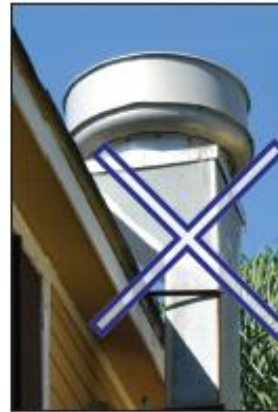
Restaurant ventilation equipment should not be mounted to the face of publicly visible elevations, nor should features like windows be removed for installation. Electric meters should not be located on the front elevation.
