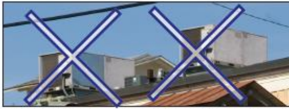
Rooftop mechanical equipment should not be installed in a visually intrusive manner.
