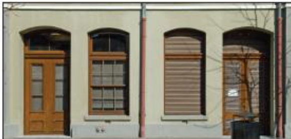
The rhythm of the storefront was maintained in the installation of the building equipment behind the louvered window and door.
