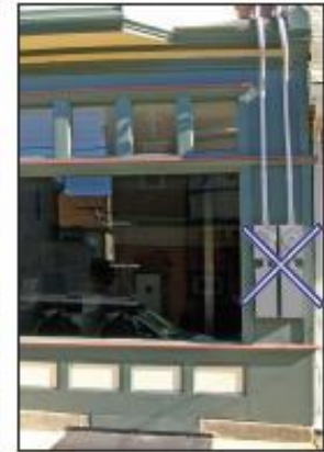
Restaurant ventilation equipment should not be mounted to the face of publicly visible elevations, nor should features like windows be removed for installation. Electric meters should not be located on the front elevation.
