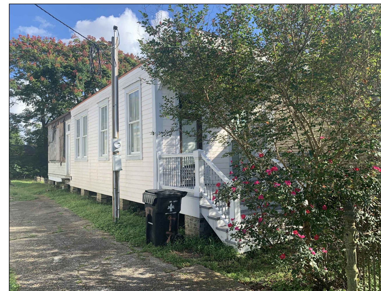
Existing Left Facade and Site
