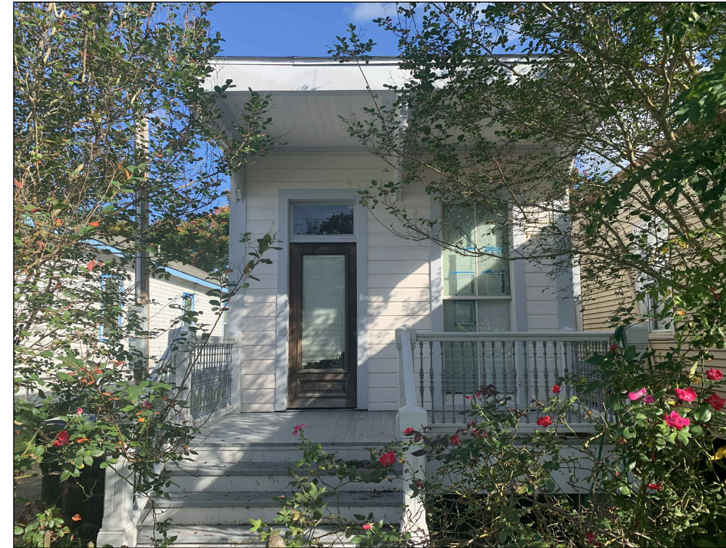
Existing Front Facade
