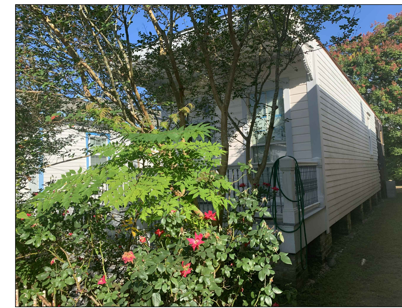
Existing Front and Right Facade
