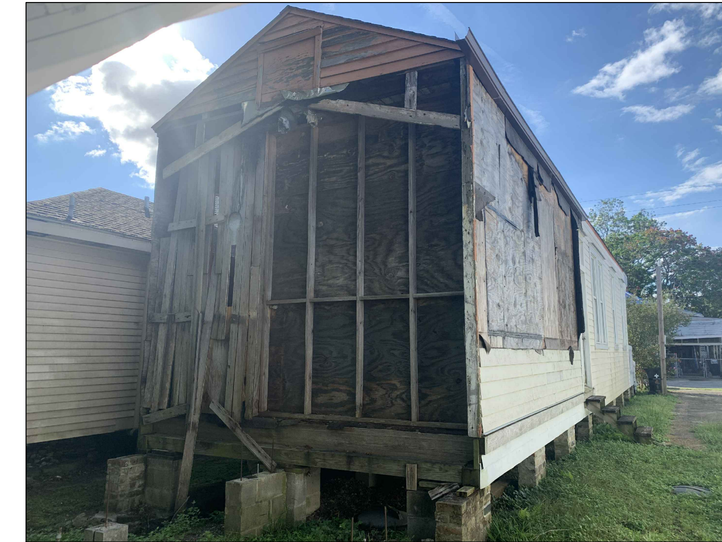
Existing Rear and Left Facades
