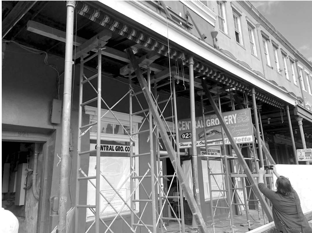
STREET FRONT FACADE WITH TEMPORARY SHORING IN PLACE.
