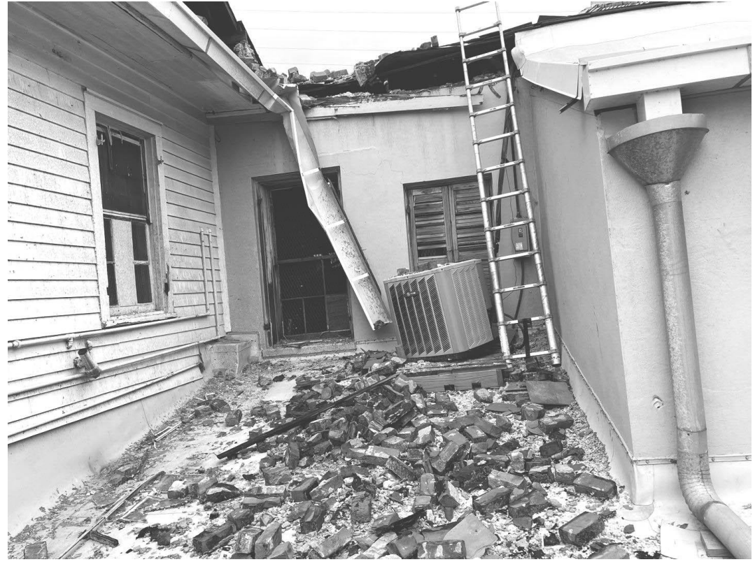
DRONE IMAGE OF BRICKS ON EXISTING ROOF STRUCTURES AND DAMAGED GUTTER.
