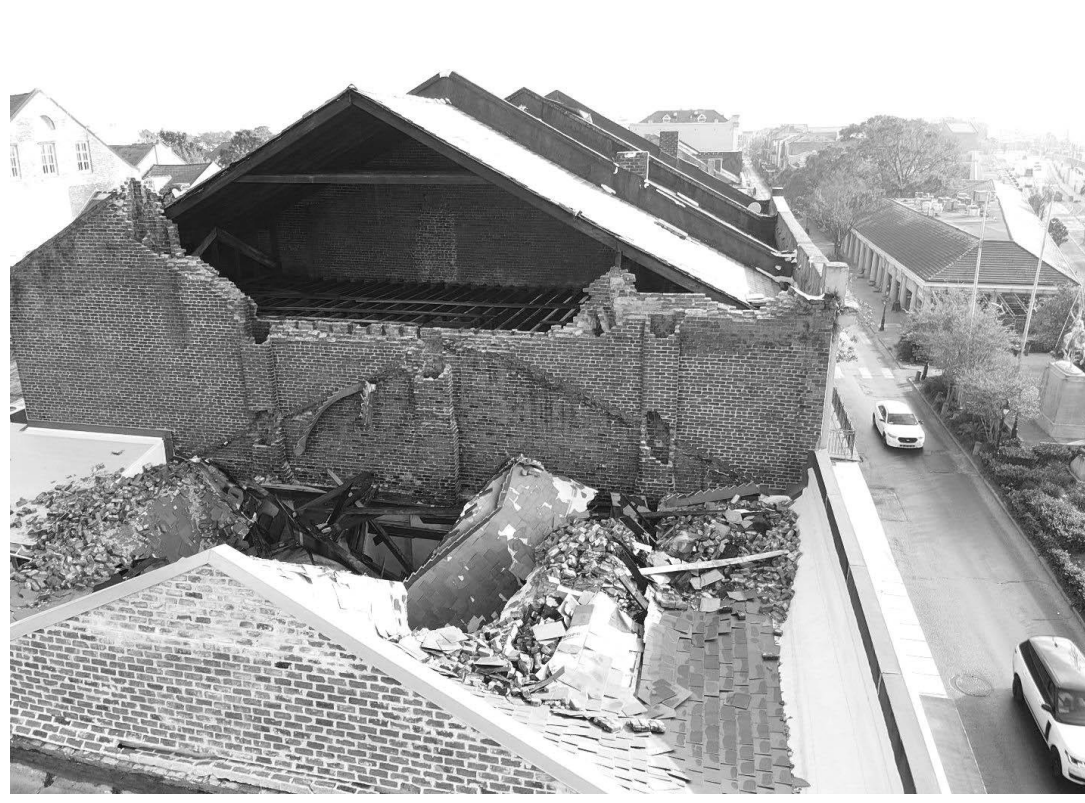
DRONE IMAGE OF COLLAPSED BRICK PARTY WALL.
