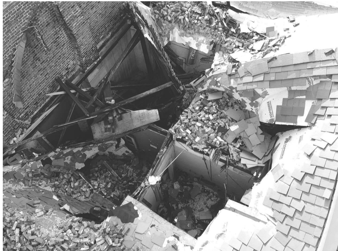
DRONE IMAGE OF COLLAPSED SLATE ROOF.
